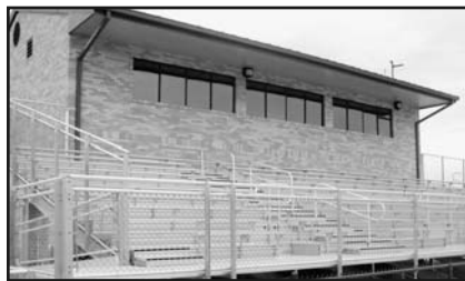
Track & Field Complex
